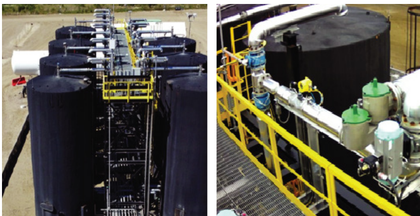
Figure 9: Tank Manway Module including vent lines & instrumentation
