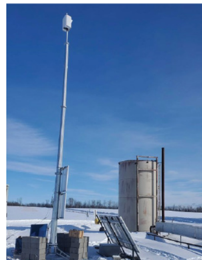
Figure 29: Kuva Camera Installation ETC 13-35 Well Site
