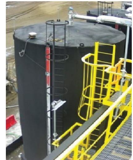
Figure 28: View of Tank Farm from West Kuva Camera
