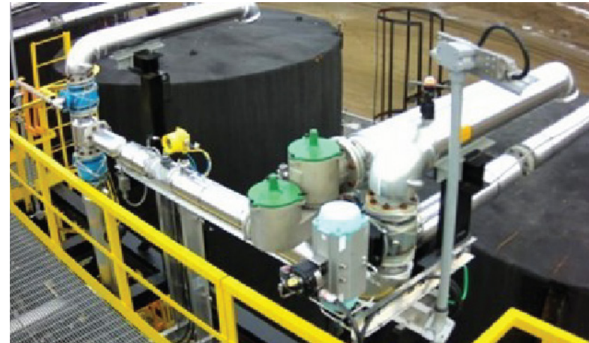
Figure 26: View of tank farm from East Kuva Camera
