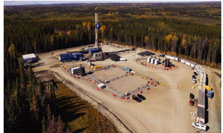
Figure 14: Tourmaline Drilling Rig Operation
